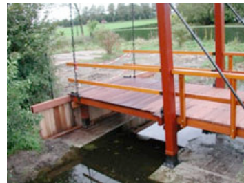
2. Sheetpiling nearby bridge in Lisse (NL)
