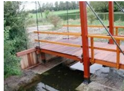
2. Sheetpiling nearby bridge in Lisse (NL)
